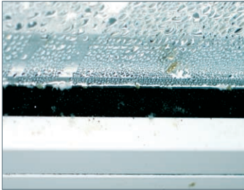
Higher risk of condensation and mould formation due to conventional aluminium spacers
